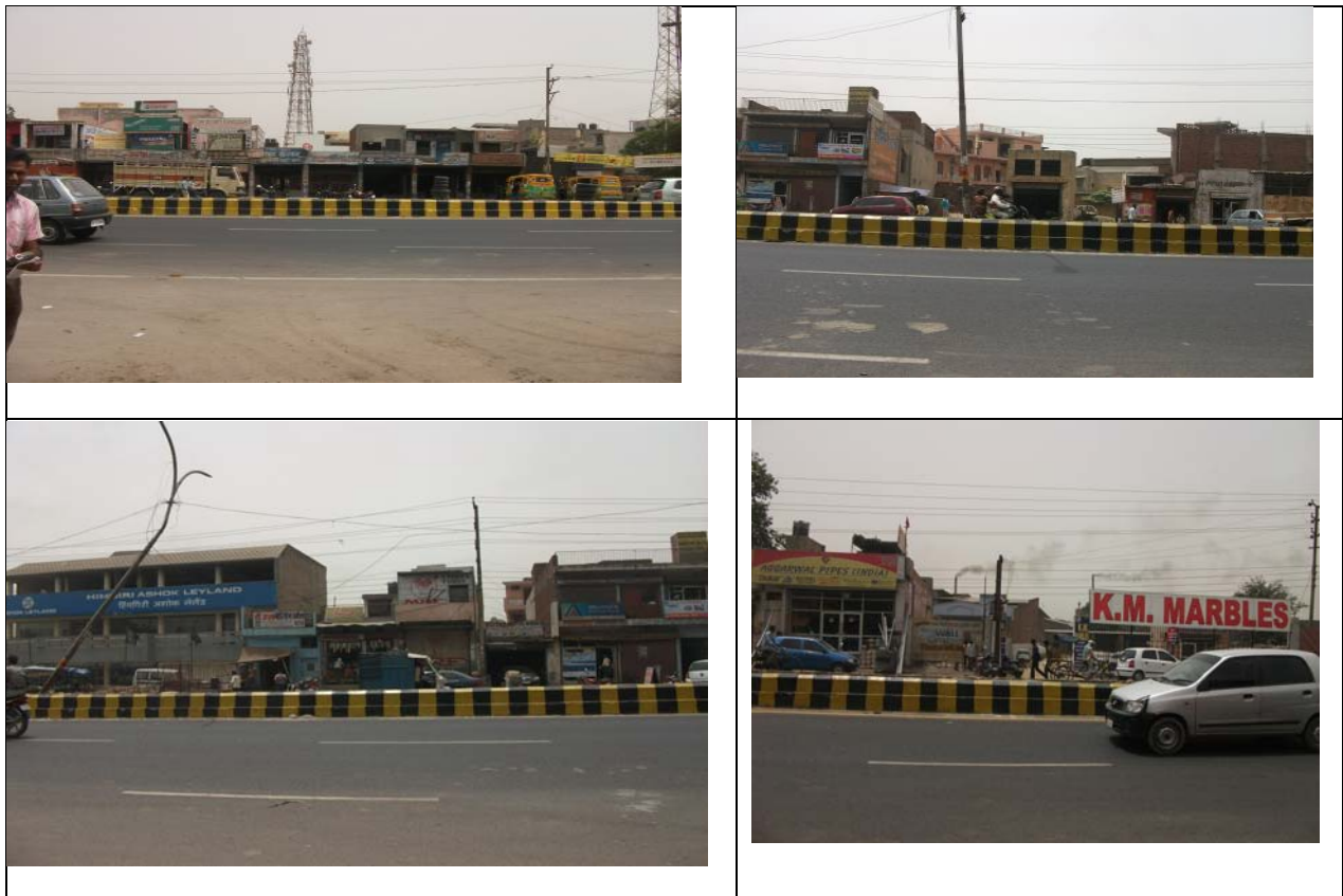
Figure 2: Partial Encroachment in RoW by Shops
