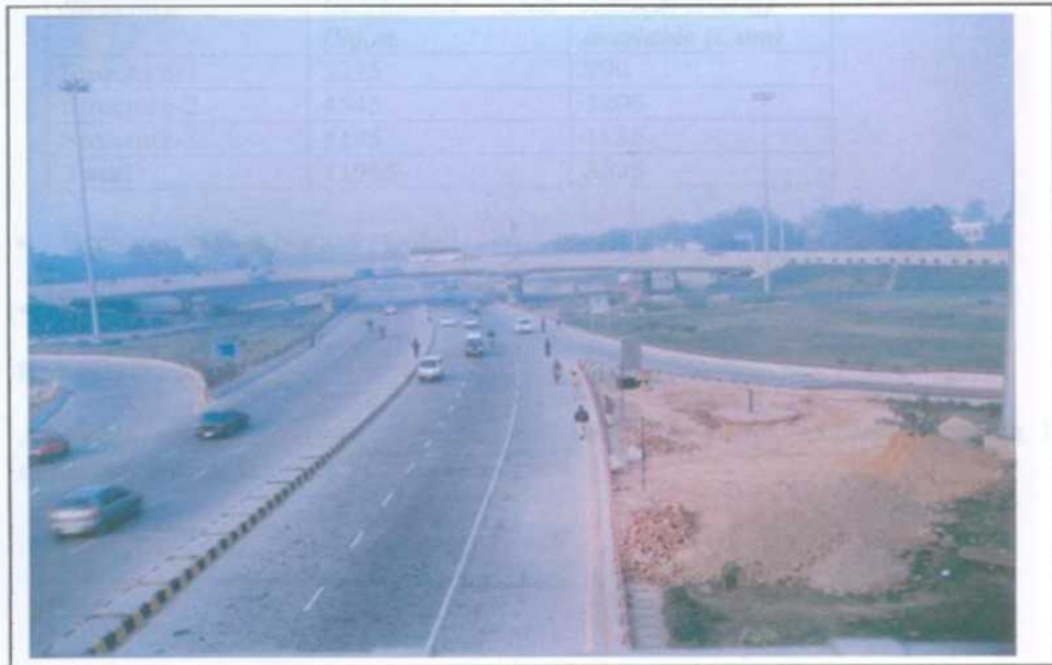
Artificial Recharge Structure at AIIMS Fly-over
